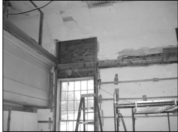
...balcony and original window height
