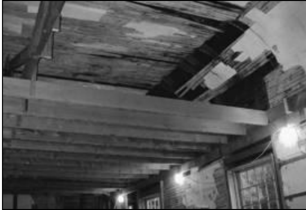
Old joists removed to reveal coved ceiling,...
