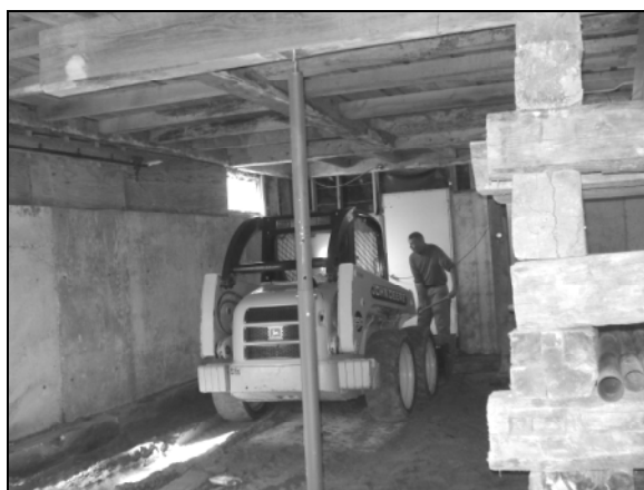
Basement floor excavated, hall floor leveled, steel beams added for support
