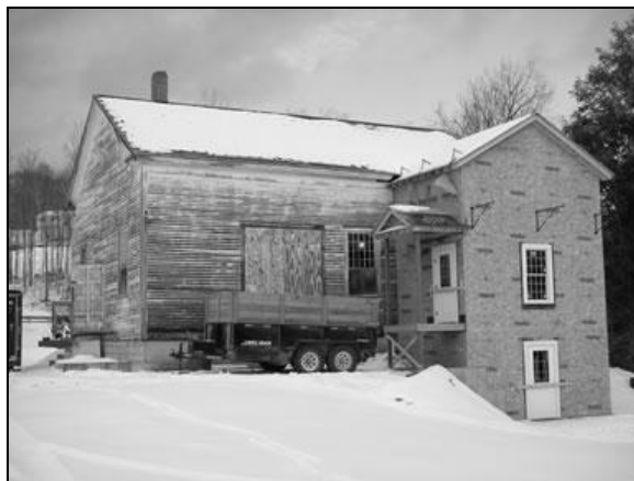
New addition on south side.
